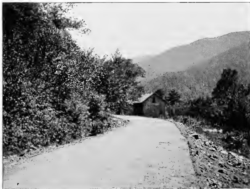
Sandstone or "bluestone" road, built in Ulster county, N. Y., by state engineer E. A. Bond, M. Am. Soc. C. E., in 1900.
